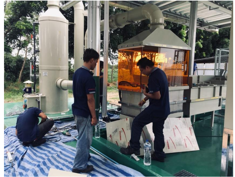
Wet Scrubber : HCL Acid
