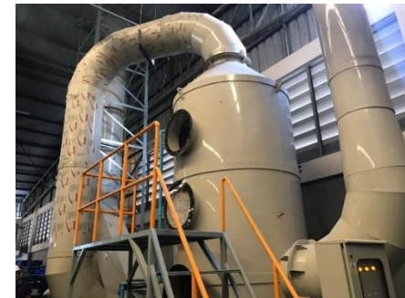
Onsite Testing /QC
