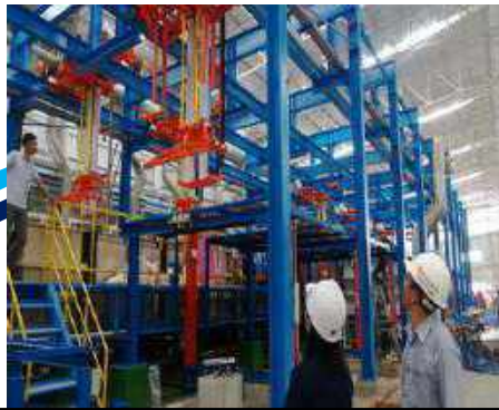
Surface Treatment Line
